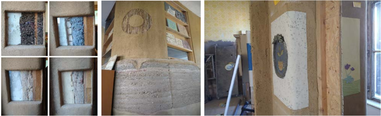
Figure 17, Figure 18 and Figure 19: Eco-centre of ArTUR is a workshop site but also a demonstration building for the NFBM (all photographs by H. Pifko).
